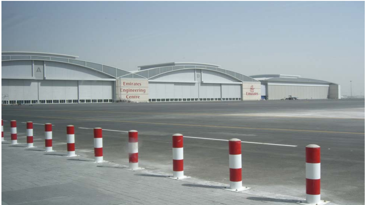
Emirates Engineering Center
